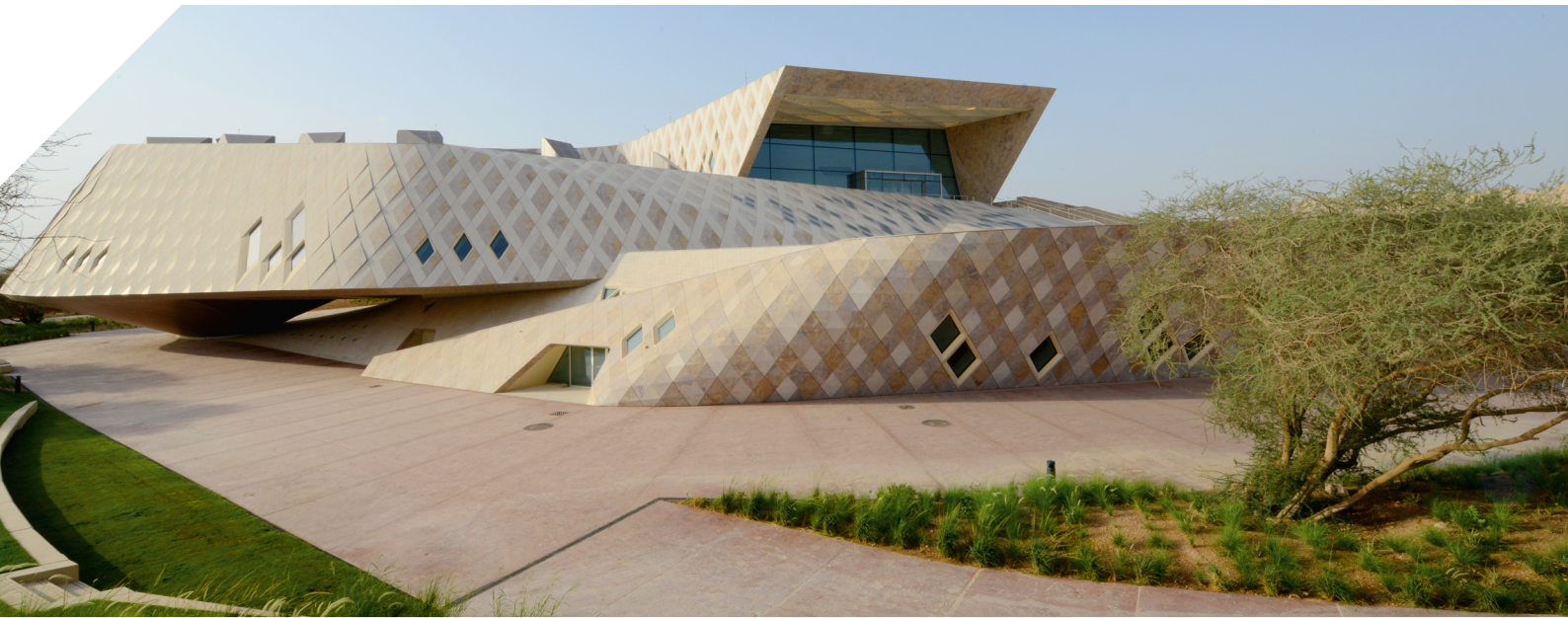
Sheikh Zayed Desert Learning Center (United Arab Emirates): building performance simulation, HVAC design optimization, simulation for LEED&BREEAM certification
