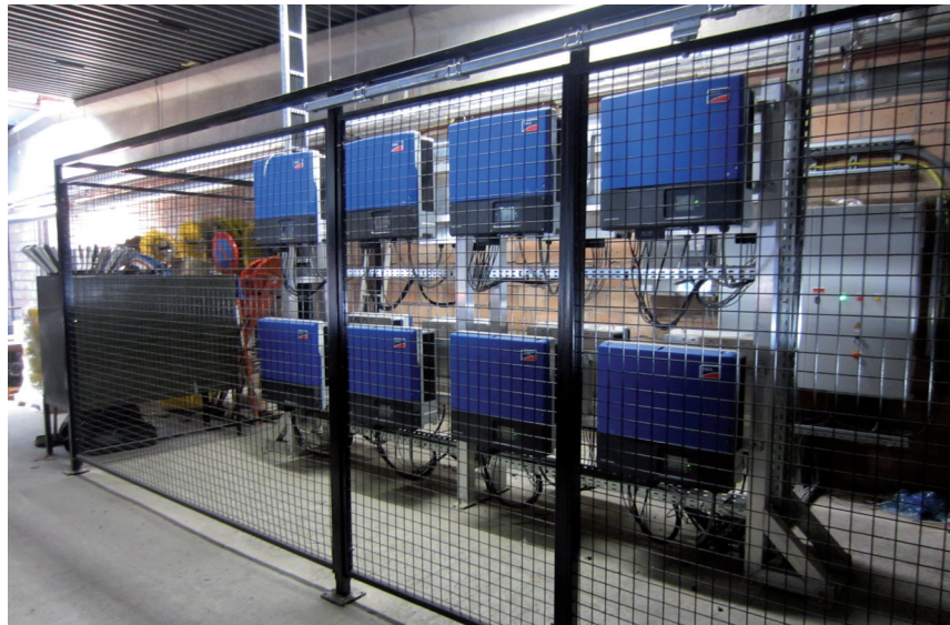
FIGURE 3: COMMERCIAL-SCALE CONTROLLABLE PV SYSTEMS ARE BUILT WITH SMA SUNNY TRIPOWER INVERTERS AND CAN BE AGGREGATED TO THE DESIRED PV PEAK POWER; THE PHOTOGRAPH SHOWS 15 INVERTERS MOUNTED BACK-TO-BACK ON A RACK AT THE MUNICIPAL WORKSHOPS
