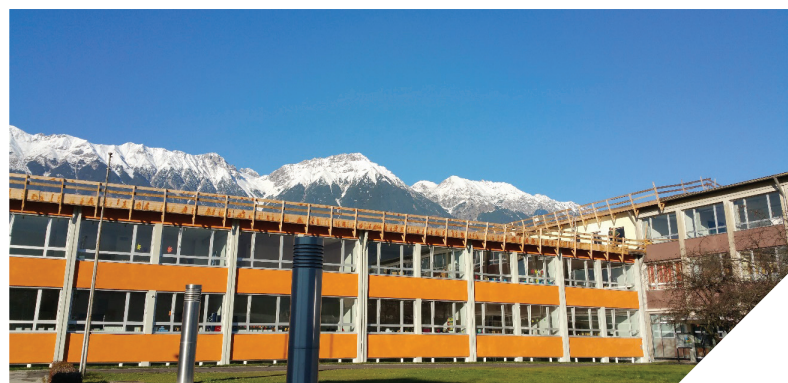
//02 School going through refurbishment, Innsbruck
